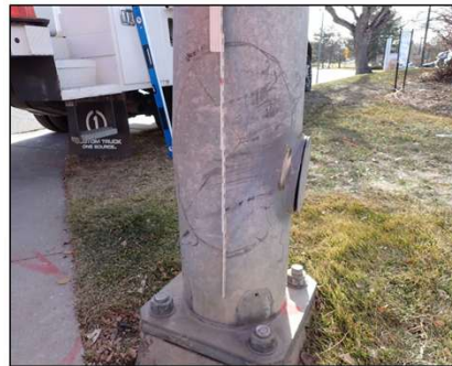
IMPACT DAMAGE IN NORTH SIDE OF COLUMN
