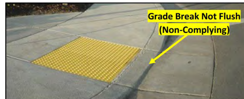
Figure 36: Non-Complying Grade Breaks
