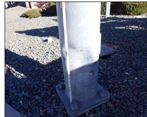
IMPACT DAMAGE ON SOUTHWEST SIDE OF COLUMN
