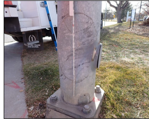
IMPACT DAMAGE IN NORTH SIDE OF COLUMN
