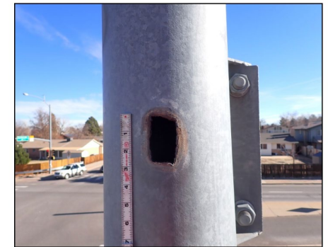
TORCH CUT HOLE IN WEST SIDE OF COLUMN ADJACENT TO UPPER CONNECTION
