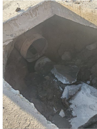
Excavated collapsed pipe
