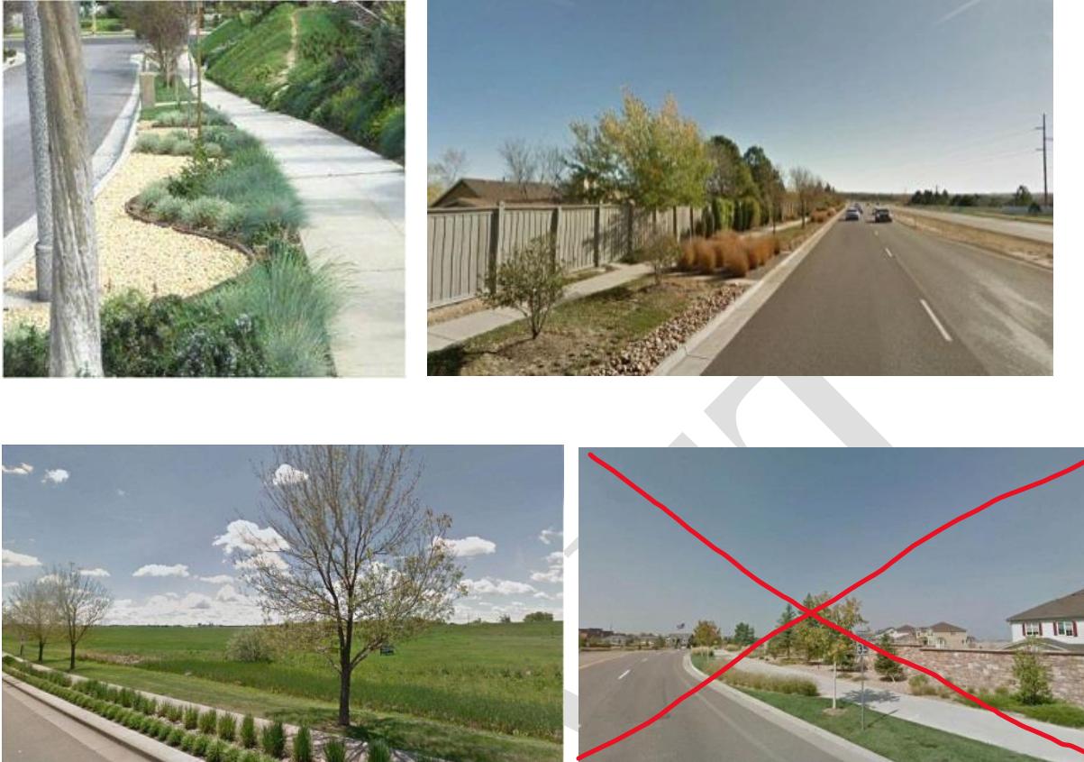
Figure 4.7-8: Examples of Detached Sidewalk Curbside Landscapes
