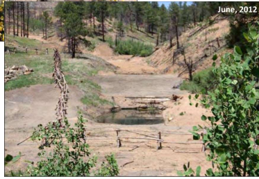
Trail Creek Post-Fire Restoration with Sediment Catchment Basin
