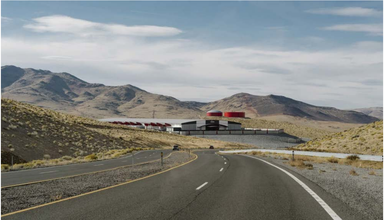
A data center run by Switch in the desert east of Reno, Nev., in 2018. Jason Henry / The New York Times / Redux Pictures
