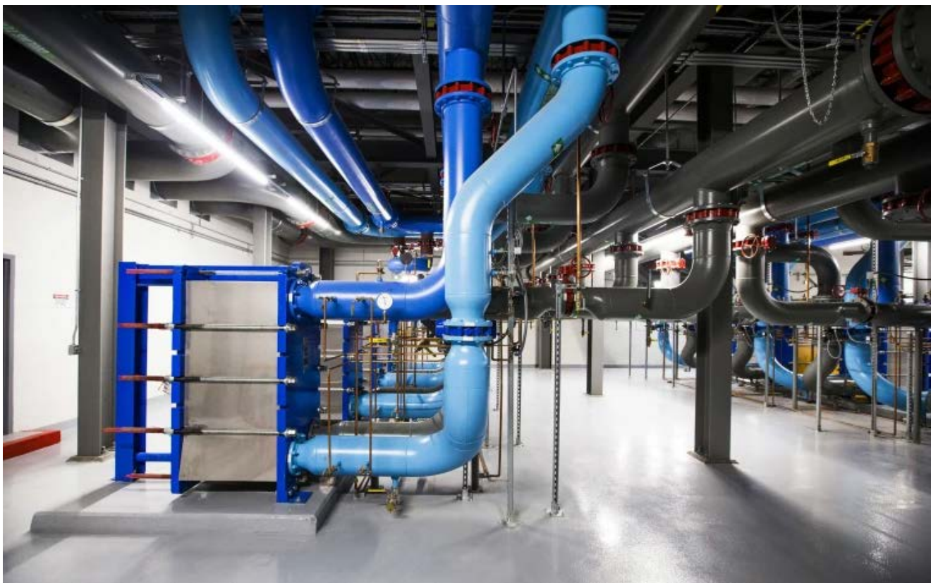
The system used to cool servers inside the Apple Data Center in Mesa, Ariz. Tom Tingle / The Republic / USA Today Network
