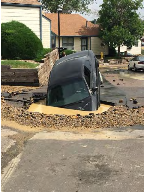
Figure 4-16 Car Stuck in a Sinkhole Caused by a Water Line Break in June of 2018
