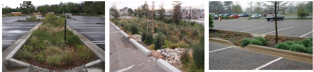
Figure 4.7-24: Parking Lot Stormwater Treatment Design
