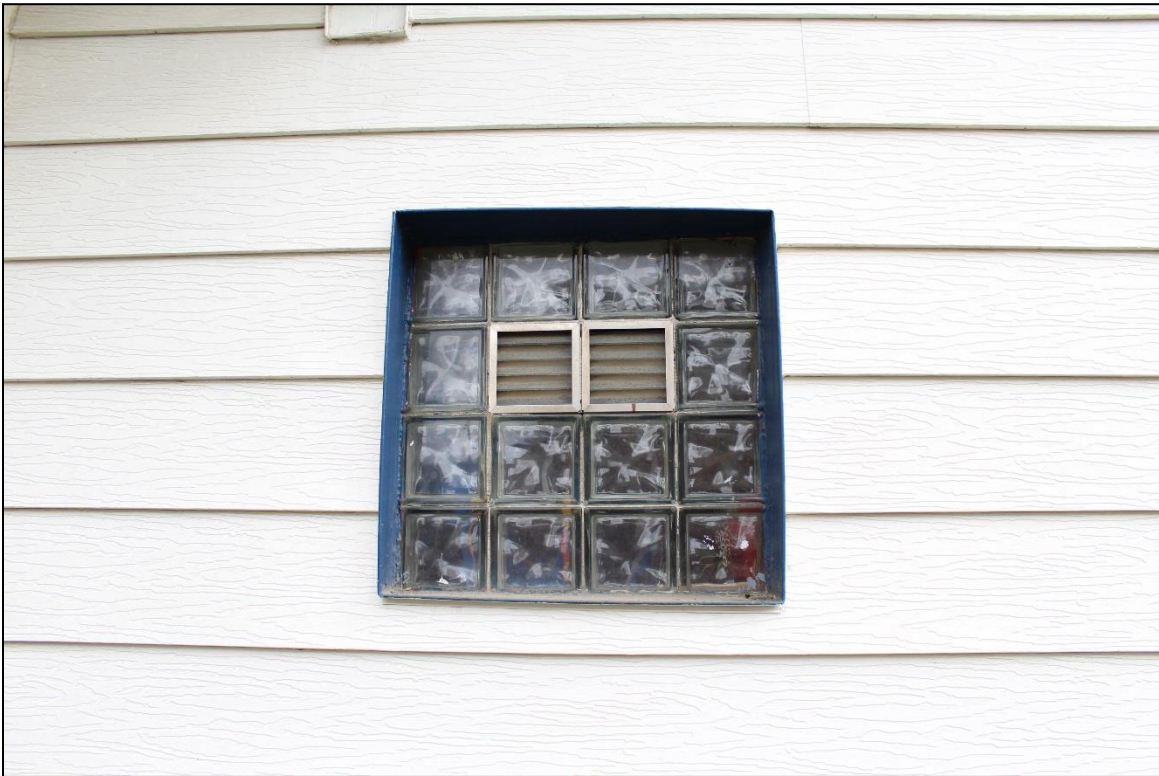
Figure 26: South elevation, glass block window. Note the aluminum frame. Facing west. Photo: Emma Lane.
