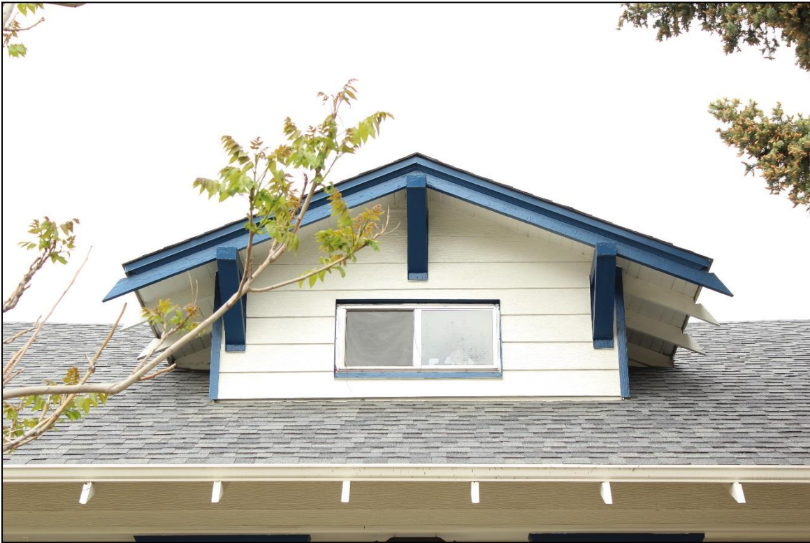
Figure 27: Façade, 2 nd floor window dormer. Facing west. Photo: Emma Lane.
