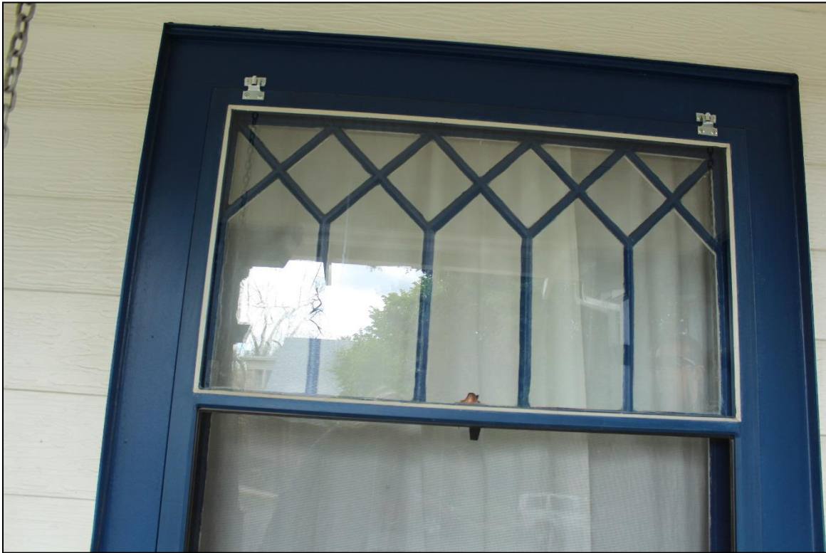
Figure 12: Façade, northern window. Note the muntins and storm windows. Facing west. Photo: Emma Lane.
