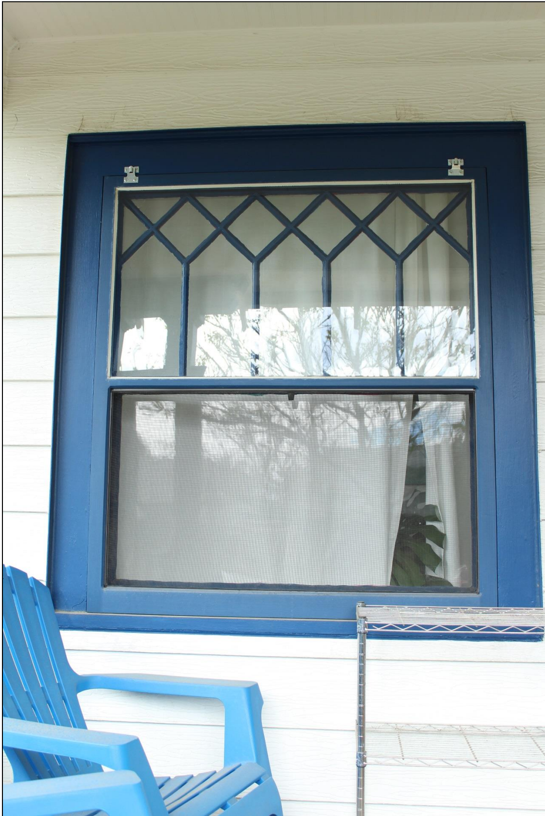
Figure 11: Façade, southern window. Note the muntins and storm windows. Facing west. Photo: Emma Lane.
