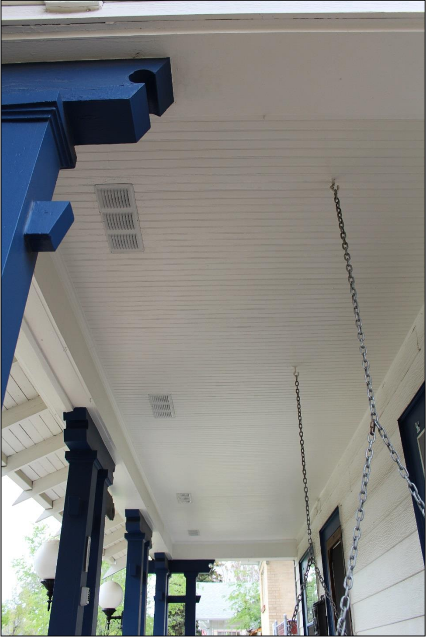
Figure 17: Façade, porch roof. Facing south. Photo: Emma Lane.
