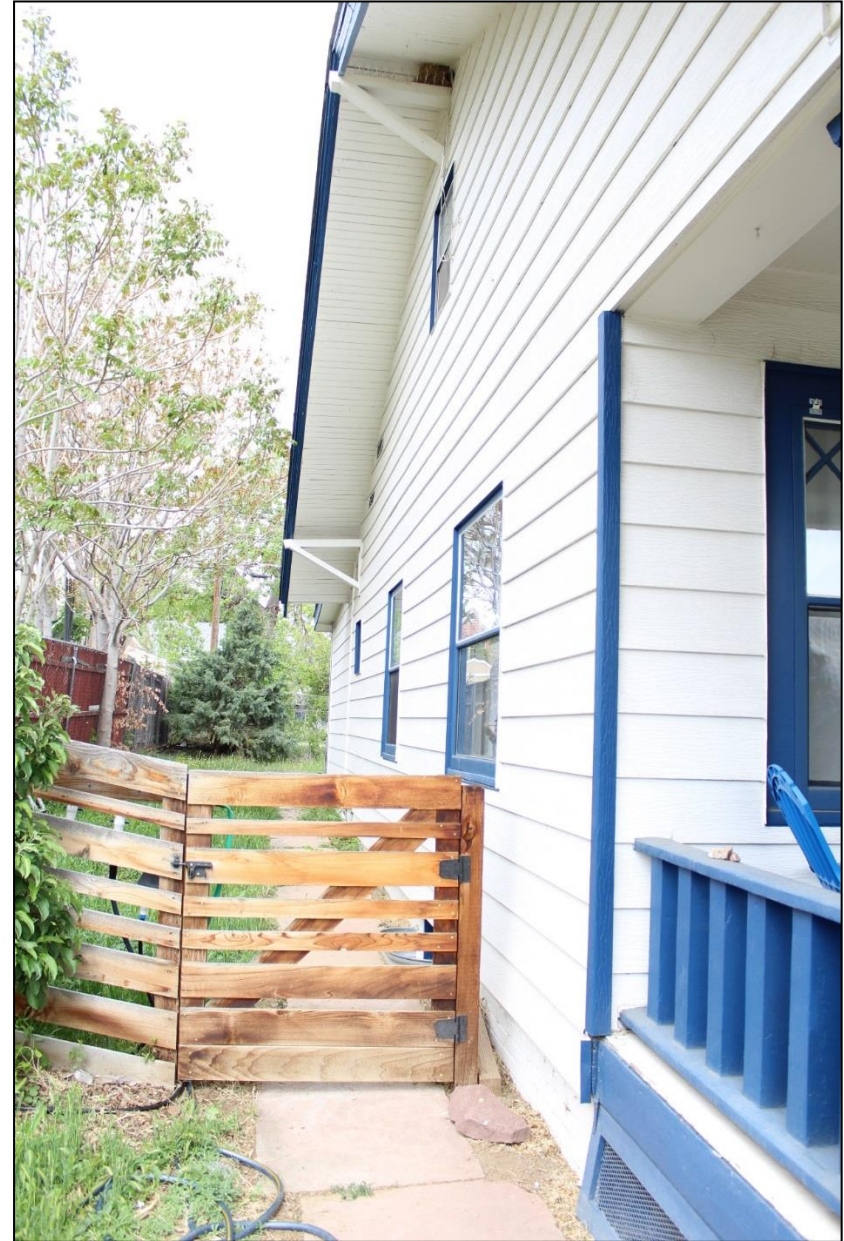
Figure 24: South elevation. Note overhanging eaves and knee brace brackets. Facing west. Photo: Emma Lane.
