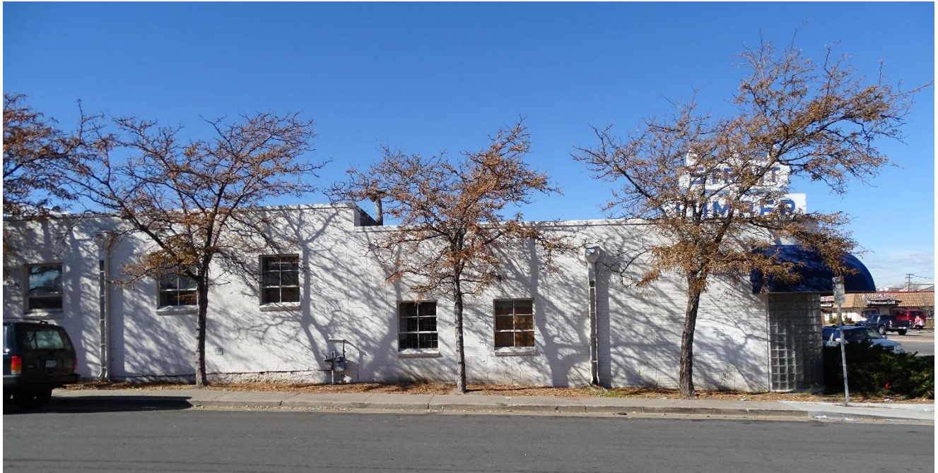
Fig. 19: Strait Lumber Company storefront and warehouse, (east elevation), 2018. Photo: Drake Brownfield.
