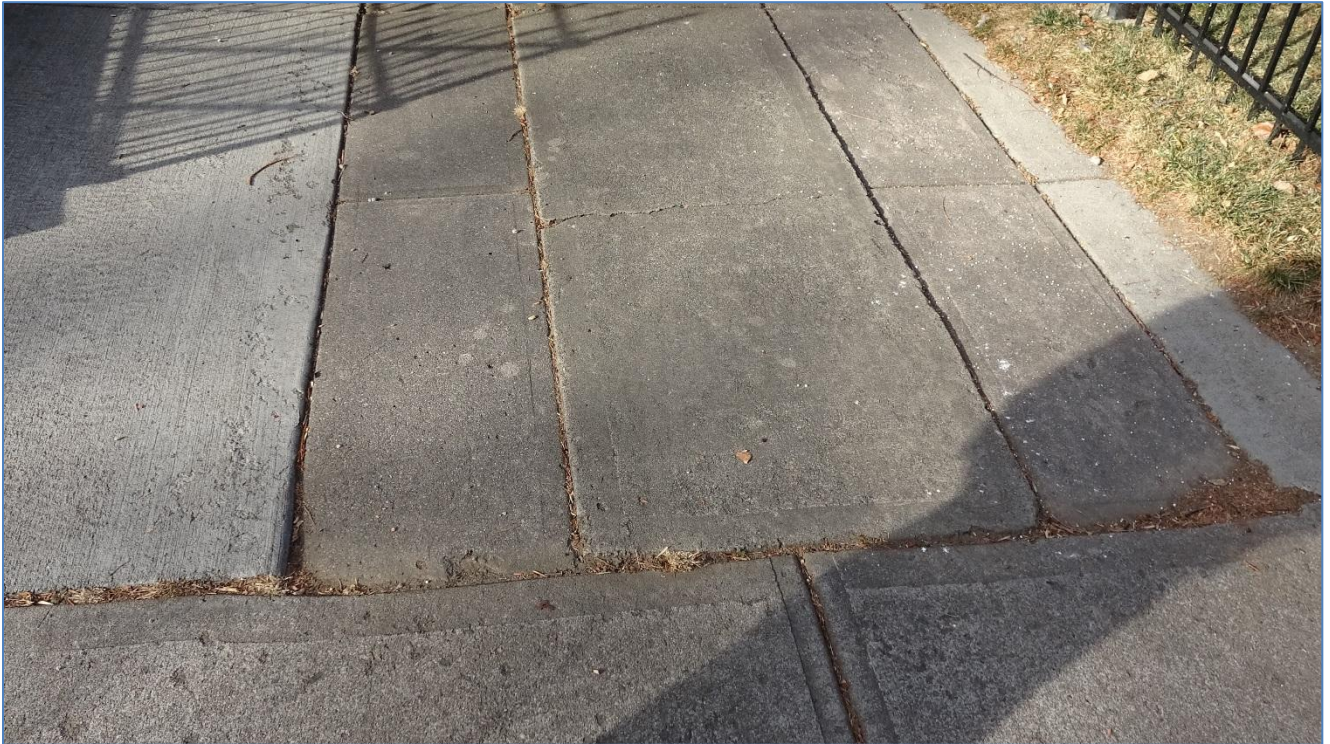
Fig. 16: Original and contemporary concrete driveway portions. Photo: Drake Brownfield, 2017
