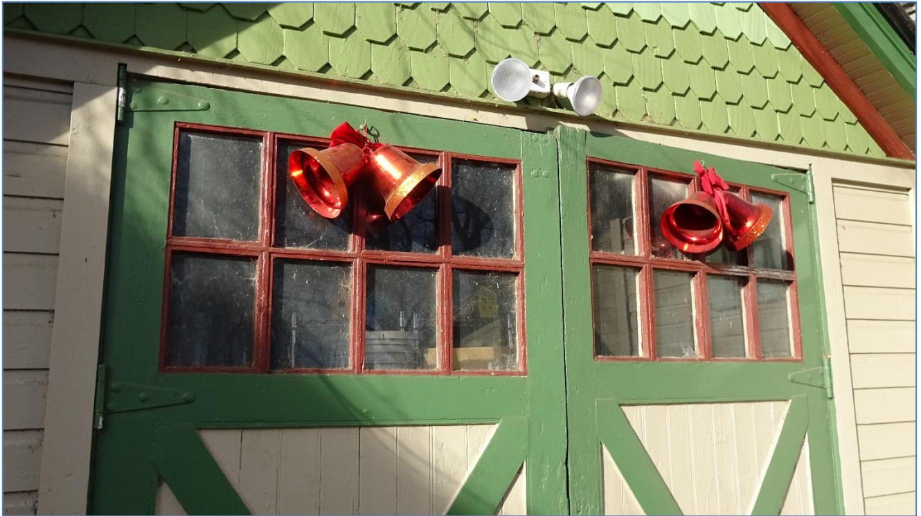
Fig. 15: Detached garage window detail. Photo: Drake Brownfield, 2017
