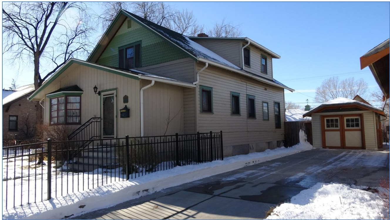
Fig. 12: North elevation. Photo: Drake Brownfield, 2017
