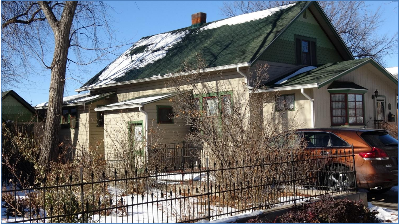
Fig. 11: Southern elevation. Photo: Drake Brownfield, 2017
