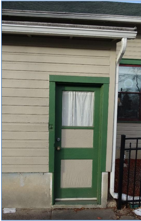
Fig. 21: South elevation, side entrance detail. Photo: Drake Brownfield, 2017
