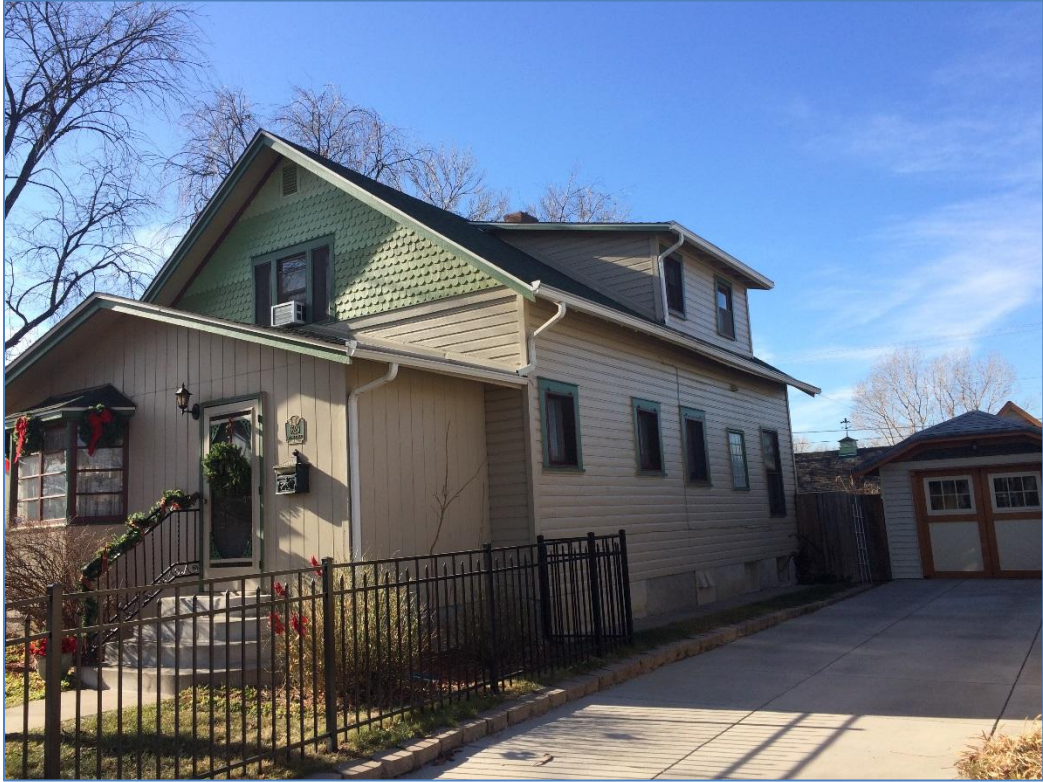
Fig. 9: Profile house shot. Front façade and north elevation. Photo: Drake Brownfield, 2017
