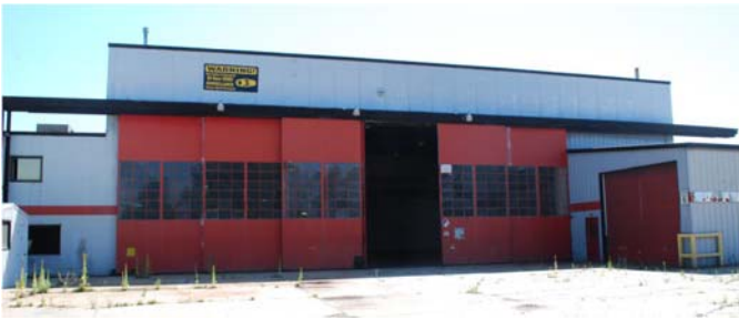
Figure 7. West Elevation hangar doors.
