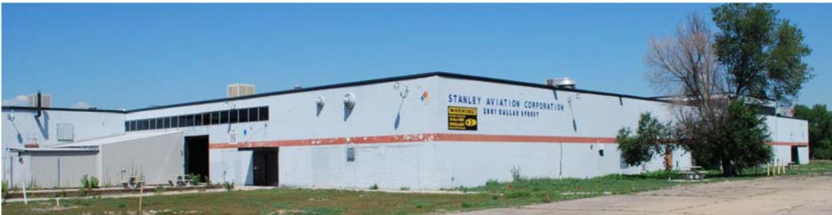
Figure 11. Southeast corner, view of courtyard area, facing northwest.
