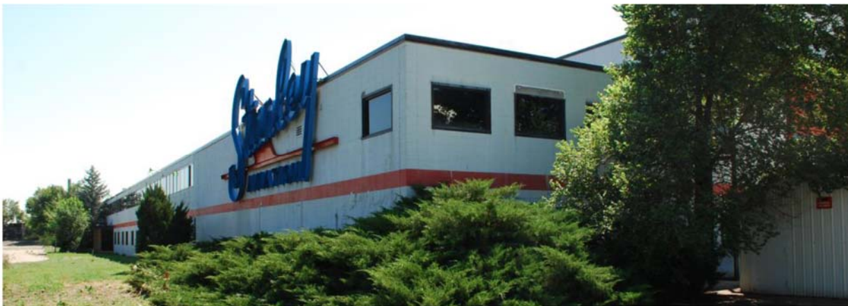
Figure 4. Northwest corner looking southeast.
