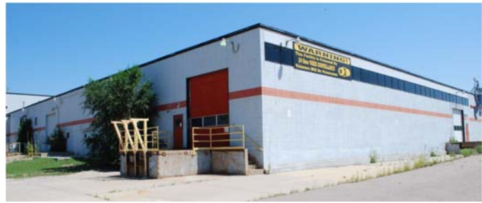
Figure 6. Southwest corner facing northeast.
