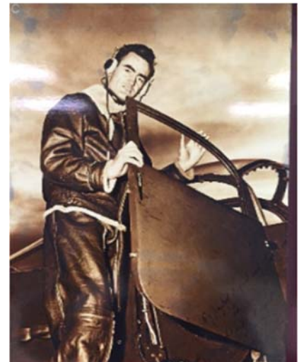
Figure 1. Pilot, engineer, & inventor, Robert M. Stanley. Courtesy of Stanley Aviation Archives.
