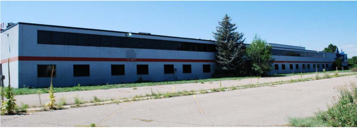
Figure 3. North Elevation looking southwest. All elevation photographs courtesy of AHSP0 8/12/2014.
