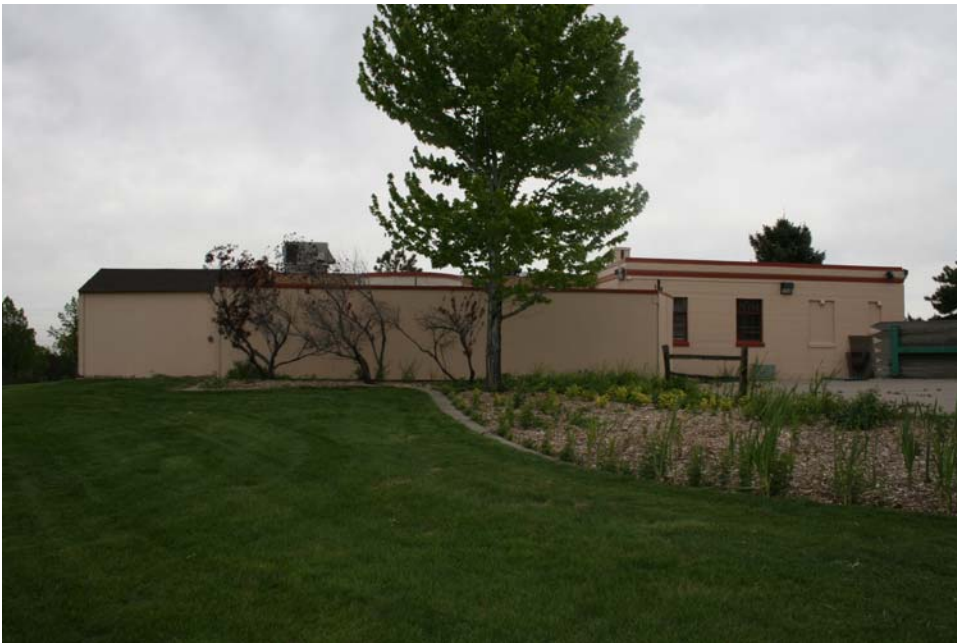
Figure 21. Bicentennial Art Center west elevation. Photograph by author.
