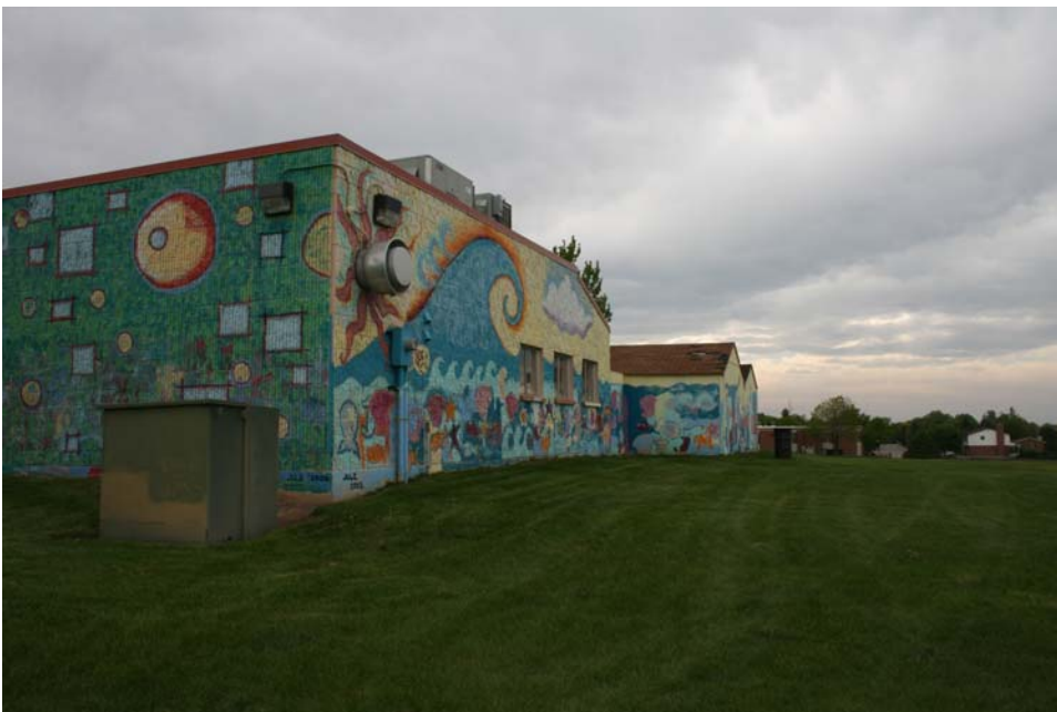
Figure 19. Bicentennial Art Center east and north elevations. Photograph by author.
