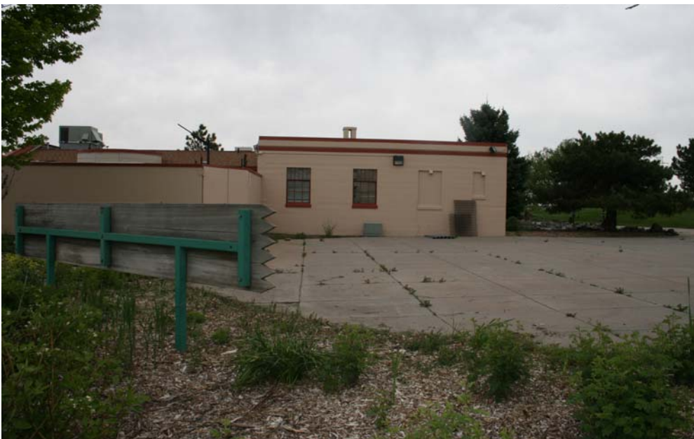
Figure 22. Bicentennial Art Center, west elevation. Photograph by author.
