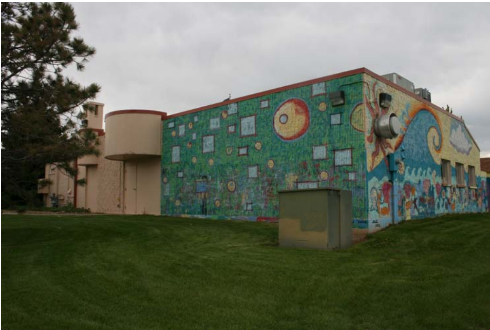
Figure 18. Bicentennial Art Center , east and north elevations. Photograph by author.
