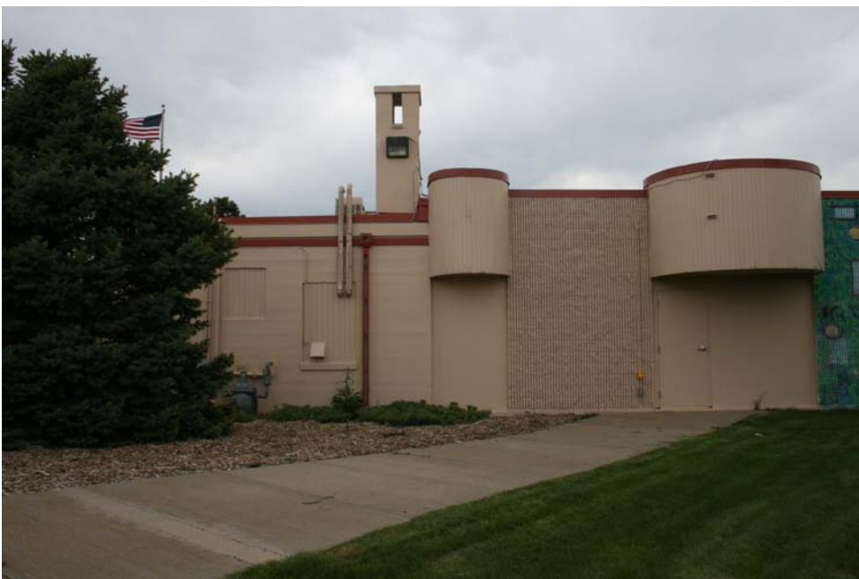
Figure 17. Bicentennial Art Center east elevation. Photograph by author.
