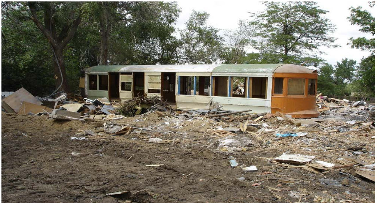
Perrott farmhouse demolished around the Trolley Trailer No. 610, July 2006.
