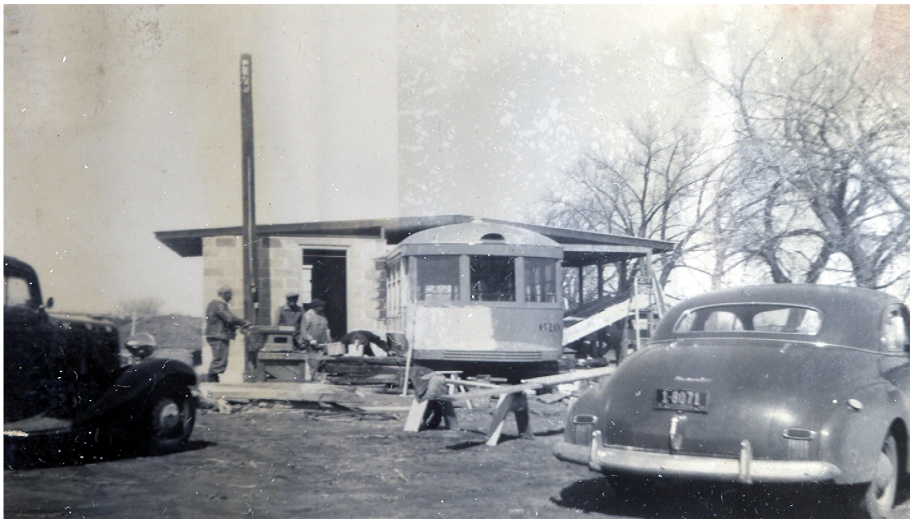
Trolley Trailer No. 610 showing Perrott farmhouse being constructed around the Trolley at the northwest corner of Colfax and Airport in east Aurora, early 1950s. (Photo courtesy- William Perrott)
