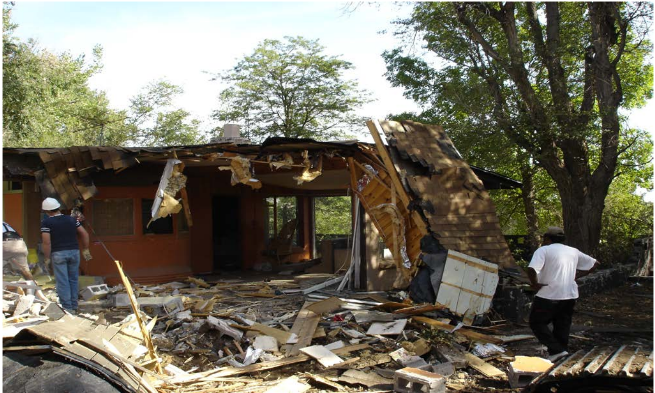
Perrott farmhouse being demolished around the Trolley Trailer No. 610, July 2006.
