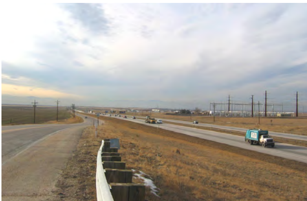
View west of the Powhatan Road overpass. Pavement, rural, and industrial land form the foreground view.
