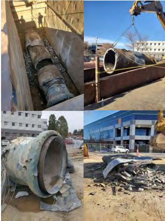
Removal – Old Pipe
