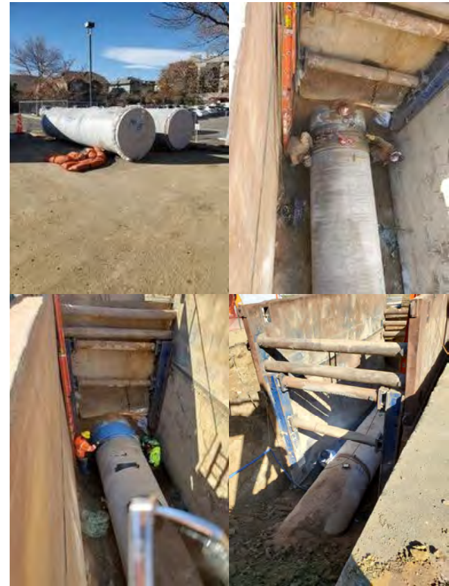
Replacement - New Pipe
